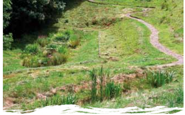
Exwick School, Exeter – a path winding through filter strips, swales, grass channels and wetlands to a pond demonstrating the wildlife and people benefits of SuDS to teachers, students and visitors.
