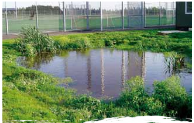
Pershore High School, Worcs – filter strips and swales play an important role intercepting silt, reducing flow rates and removing over 80% of pollution before allowing water to enter this pond. Photo: Bob Bray
