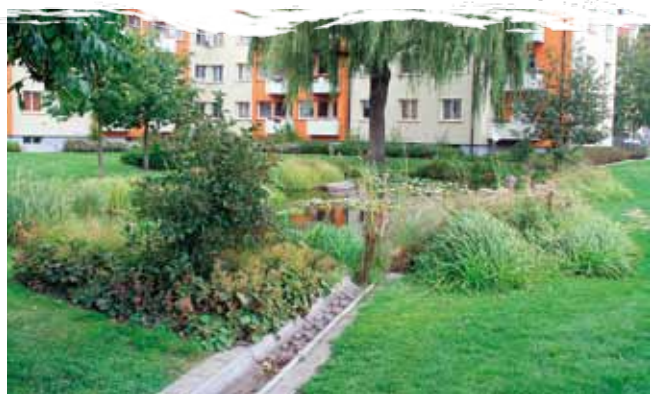
Augustenborg, Malmo, Sweden – an open channel leading from an unfenced amenity pond in a housing retrofit SuDS scheme. Photo: Bob Bray
