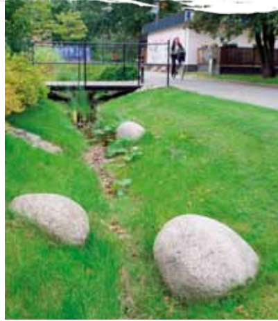
Augustenborg, Malmo, Sweden – an open swale next to a cycle route with large boulders common in many Swedish landscape designs showing a confident approach to risk. Photo: Bob Bray
