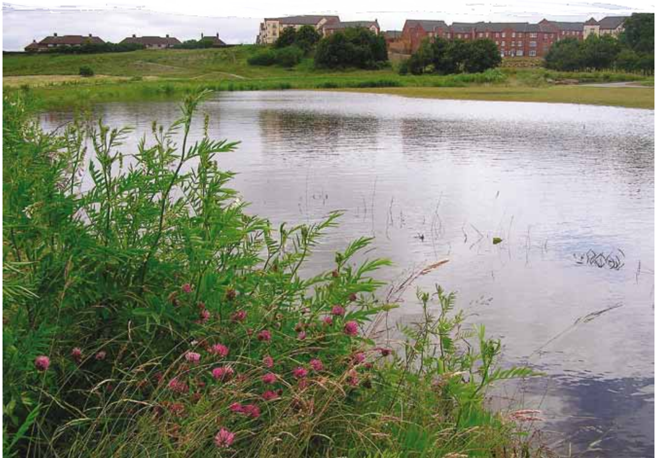
Manor Park Sheffield – under-drained sports and playing fields, the 1 in 100 year storage feature, two-thirds full at the beginning of the week in the 2007 floods but with football played on the Friday – a multi-use amenity space. Photo: Roger Nowell
