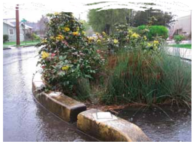
Portland, Oregon, USA – SuDS can be incorporated into street landscaping to filter oils and pollutants as well as to attenuate rainfall. Photo: Dusty Gedge
