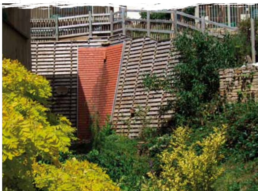
Springhill Housing, Stroud – water is kept at the surface wherever possible as with this tile hung cascade demonstrating both visual and cost benefits compared with a conventional 4m 'drop manhole'. Photo: John Day (rspb)
