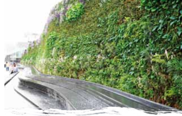
Westfield Shopping Centre, Shepherd's Bush, London – living walls help cool, insulate, reduce noise, trap airborne pollution and provide habitat for bats, birds and insects. Photo: Gary Grant
