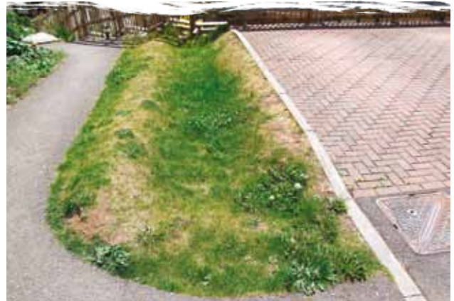
Springhill Cohousing Stroud – permeable paving and adjacent under-drained swale help trap and filter polluted water. Photo: John Day (rspb)
