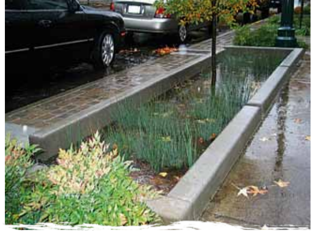
Portland, Oregon, USA – bioretention areas filter polluted road run-off, provide urban wildlife habitat and reduce local flooding. Photo: Dusty Gedge
