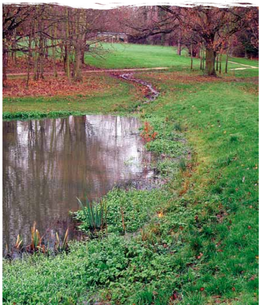
A low flow channel and linear wetland provides connectivity to a detention pond for clean runoff at the beginning of this management train. Photo: Bob Bray
