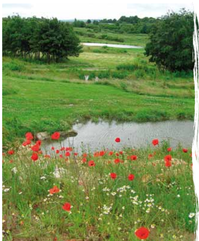
Manor Park, Sheffield – the first of three basins in the foreground collecting runoff from 300 houses with a sports arena/detention basin in the distance inundated during the 2007 floods. Photo: Roger Nowell
