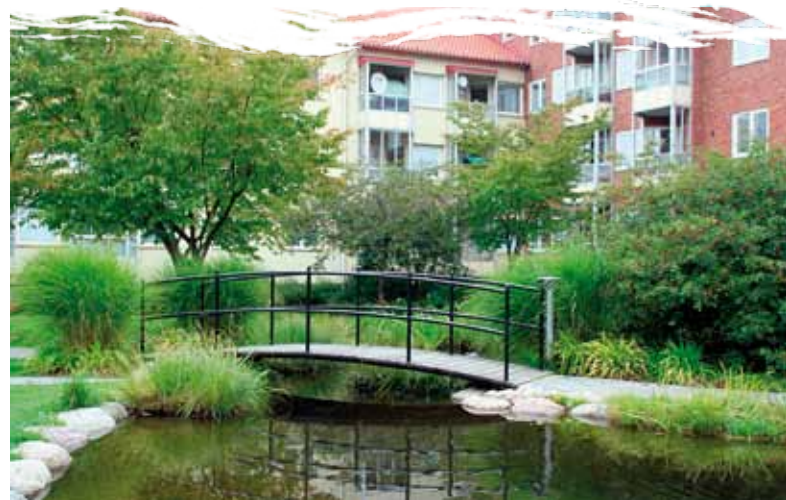
Augustenborg, Malmo, Sweden – an open water SuDS feature in a housing retrofit scheme collecting rainfall via a disconnected downpipe. Photo: Bob Bray
